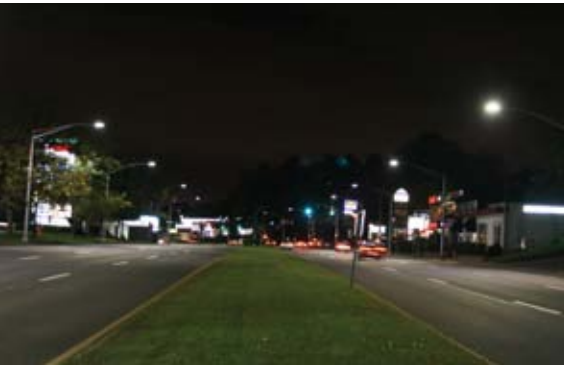
Yonkers, NY Street Lighting
