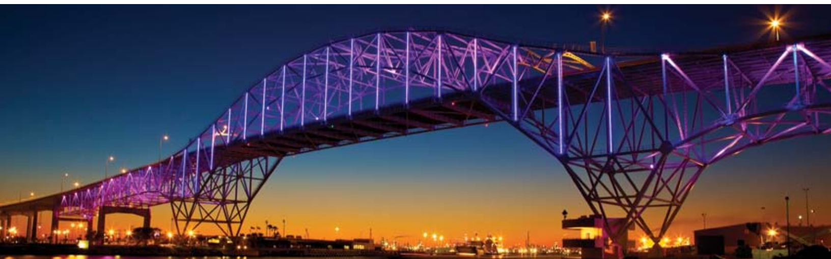
Corpus Christi Harbor Bridge, TX
